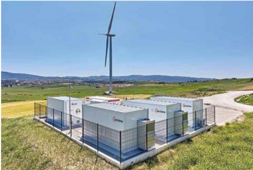
Acciona Energy installed a 1.7MW peak-power lithium-ion battery experimental facility in September 2017 at its 15MW Barasoain wind plant in the Navarre region, Spain
